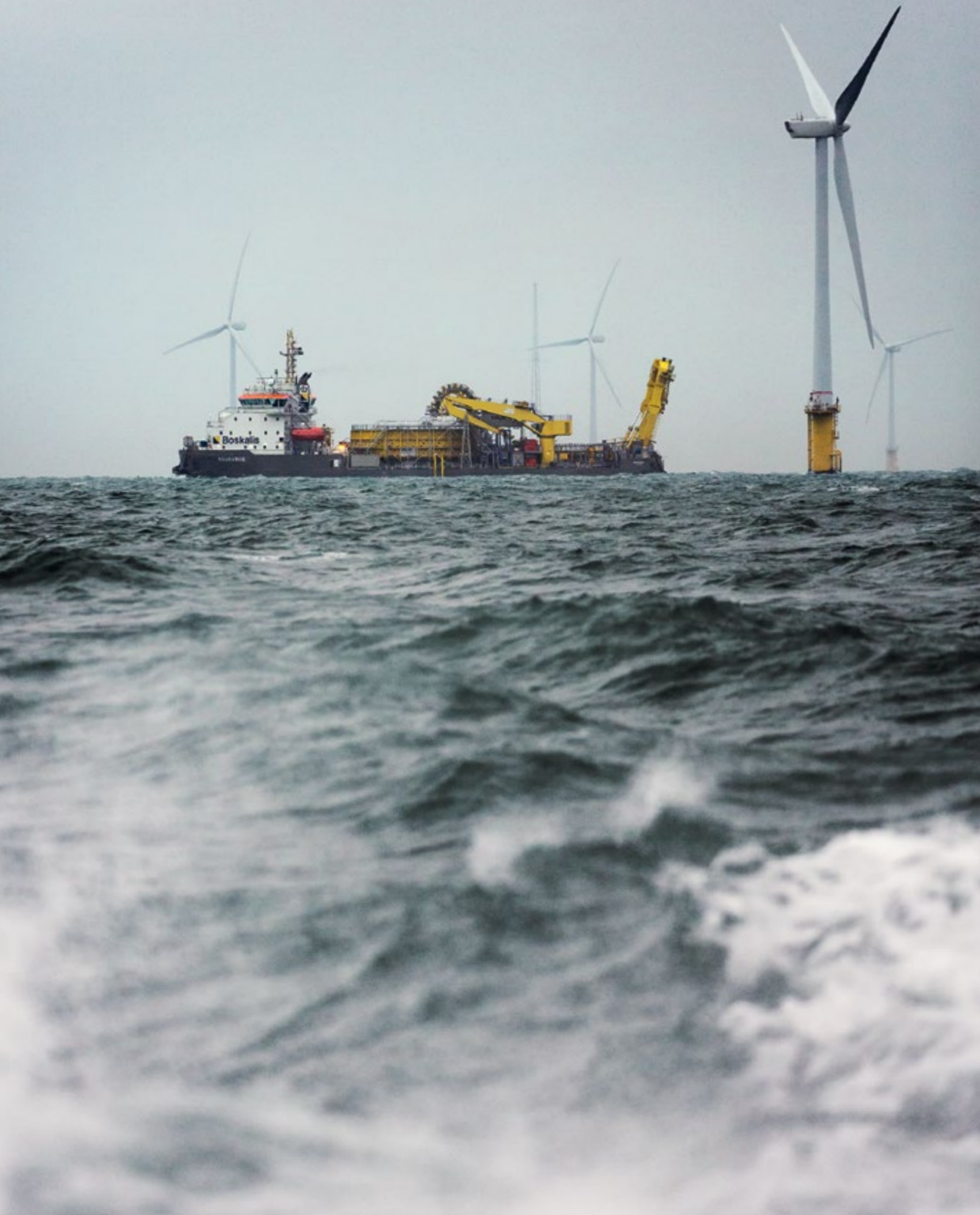
The cable-laying vessel Ndurance at work off the Dutch coast near Egmond aan Zee.
