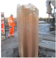
The system is used on location where very soft soil exist and a solution with PVD and surcharge is not capable to provide the required stability or residual settlement within the given construction period
