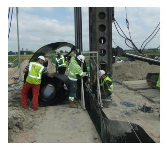
Fig. 7. Installation of the panel in partially hardened diaphragm wall (www.bam.nl).
