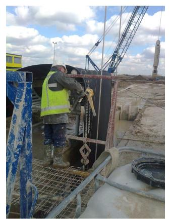
Fig. 12. Installation of the HDPE screen in the cement-bentonite wall.
