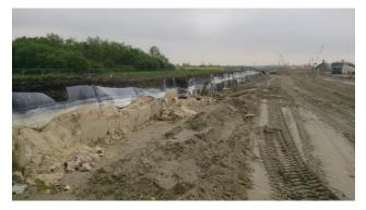
Fig. 9. The wall after installation and excavation of the installation berm.
