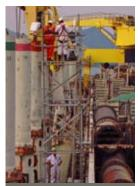
Safety tops the agenda – scaffolding is erected for all jobs, including minor work, such as the inspection of a sensor above a bottom door cylinder.
