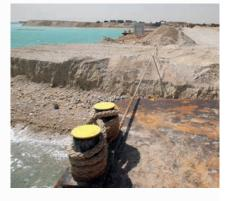
Snapback zone: if a line snaps, the sand dike will absorb the impact.
