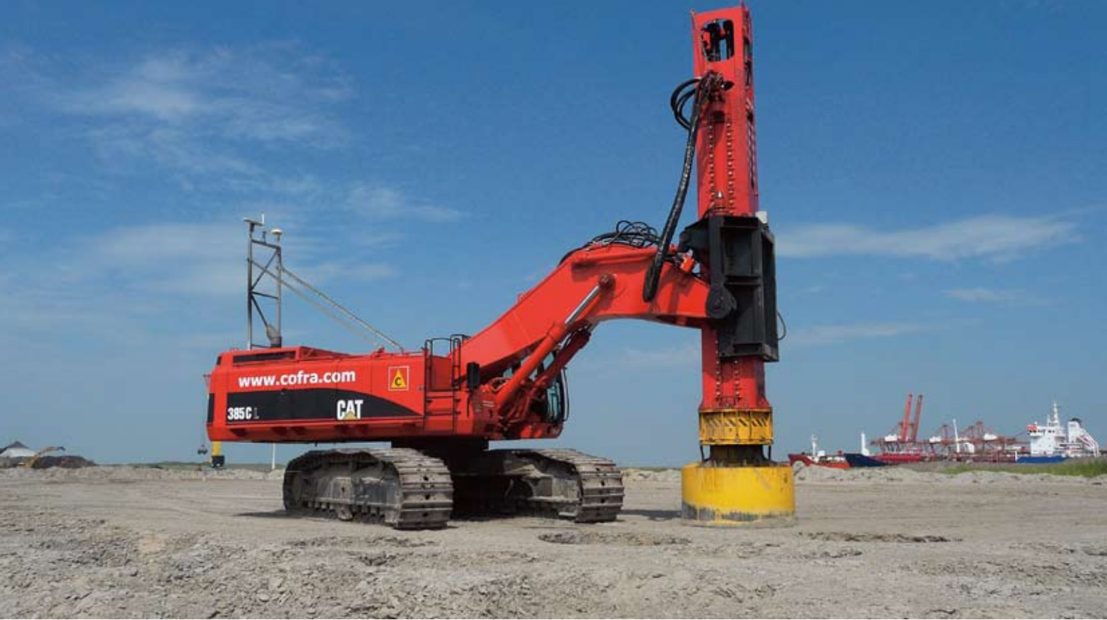
Compaction at the Vopak terminal site
