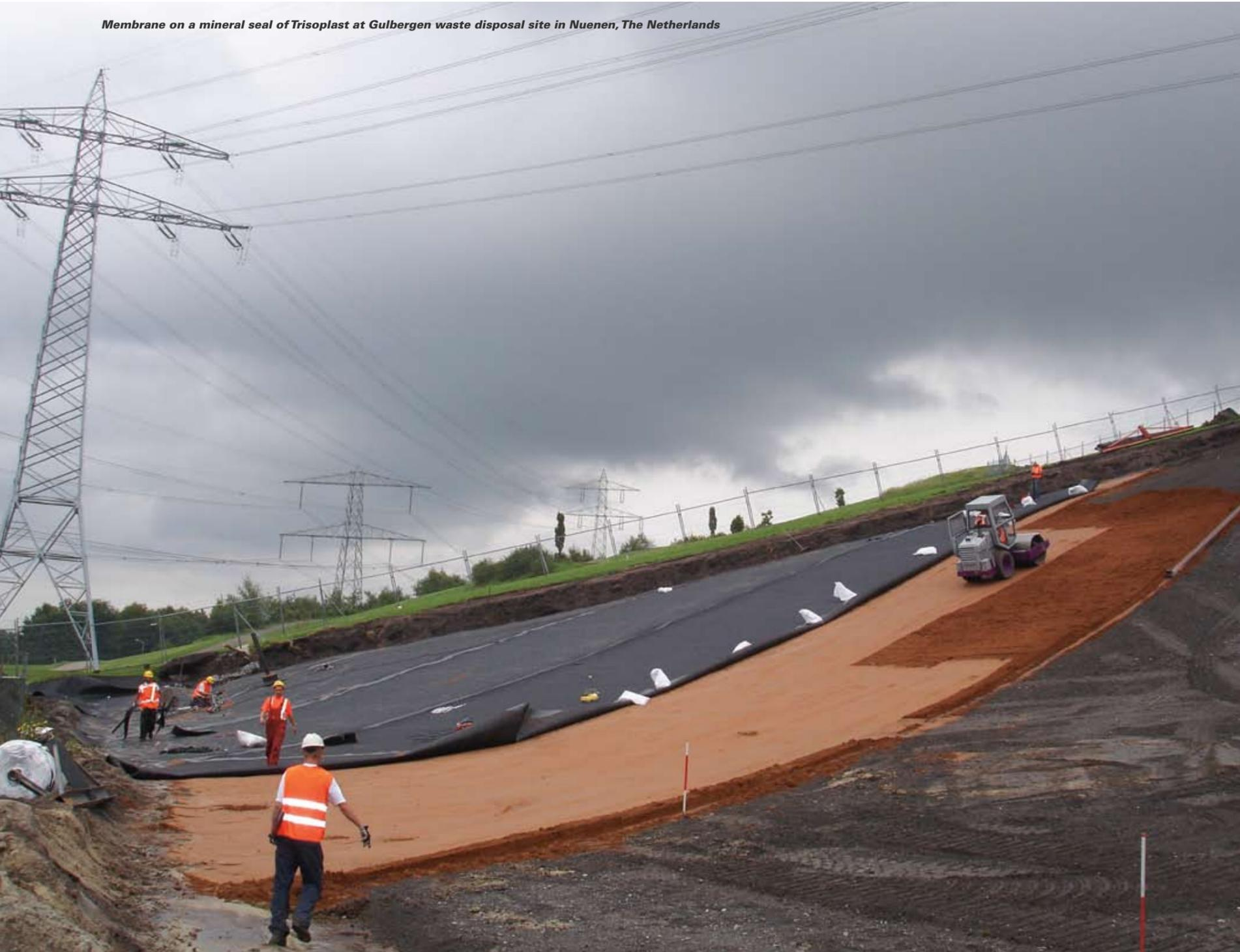
*Membrane is being unrolled with the aid of a bearing-mounted spreader*
