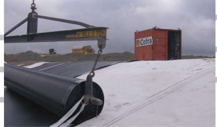
*Membrane on a mineral seal of Trisoplast at Gulbergen waste disposal site in Nuenen, The Netherlands*
