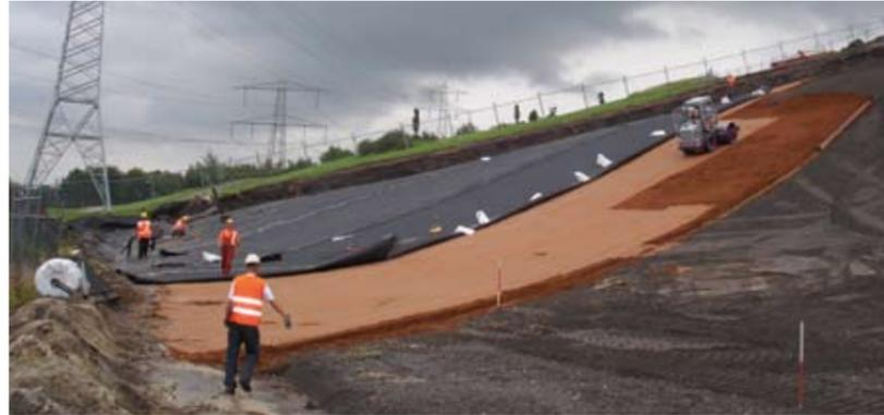
Cofra specialises in the incorporation and application of HDPE synthetic liner. Cofra is the Netherlands' largest installer of HDPE liner at waste disposal sites and in civil engineering projects. Furthermore, Cofra was the first contractor to be certified for the incorporation of synthetic liner according to the KIWA BRL K537 standard. For more than 25 years, installation crews have carried out all types of work according to the highest quality standards.
