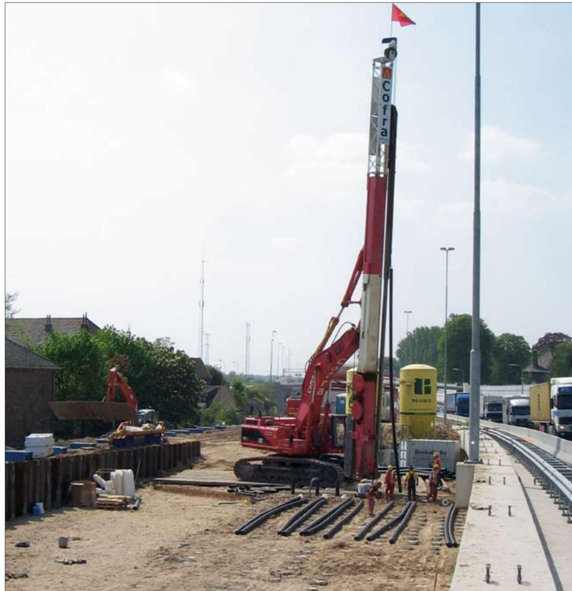
Installation of AuGeo piles for the southern carriageway of the A15, The Netherlands
