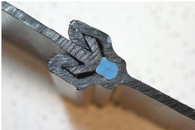
Fig. 2. Lock with Hydrotite swelling cord in swollen condition.
