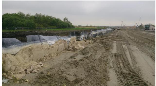
Fig. 9. The wall after installation and excavation of the installation berm.
