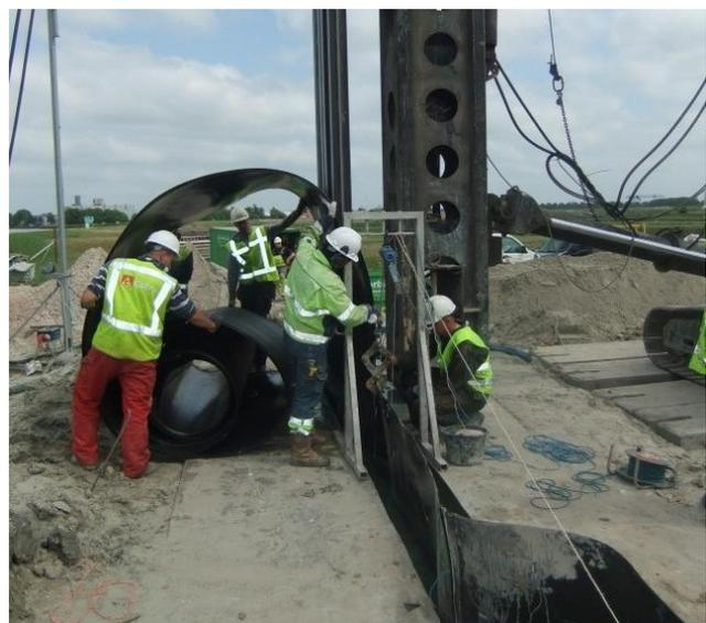
Fig. 7. Installation of the panel in partially hardened diaphragm wall ([www.bam.nl](http://www.bam.nl)).
