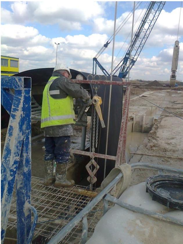
Fig. 12. Installation of the HDPE screen in the cement-bentonite wall.
