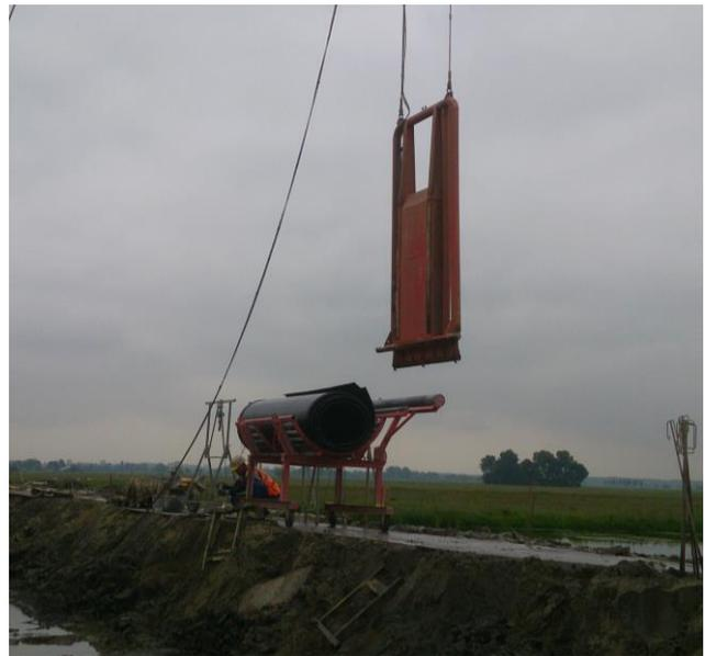
Fig. 10. Weight used for the installation of the panels top.
