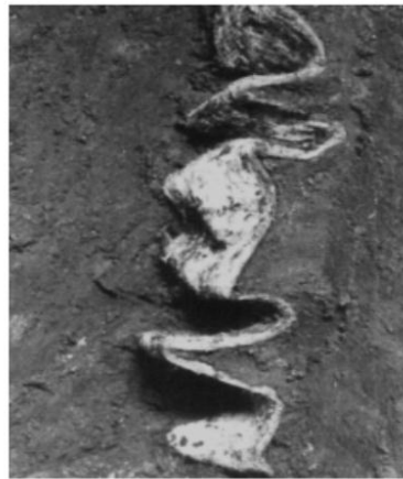
Figure 1. Drain in buckled conditions after consolidation in peat as shown in the EN 15237
